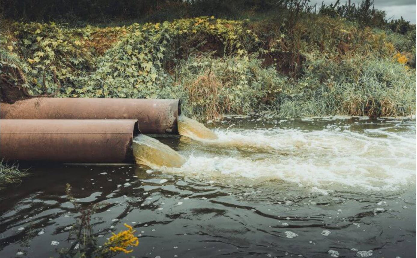
Image 28: Combined sewer overflow. Source: Shutterstock
