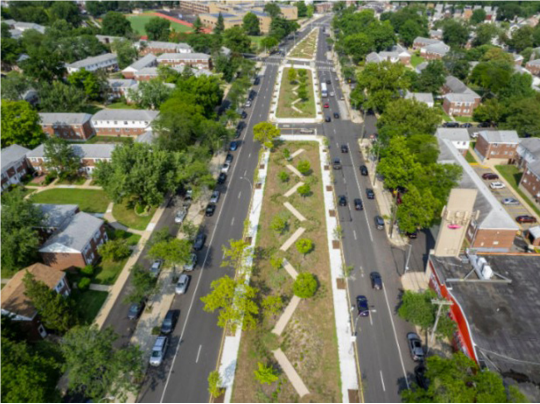
Image 25: Green infrastructure medians at Martin Van Buren High School, New York. Source: NYCDEP
